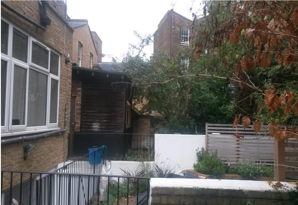
Photo 7: View of the 2 storey existing rear extension at basement and ground floor level and lightwell to basement level to adjoining neighbour No.358 Caledonian Road.
