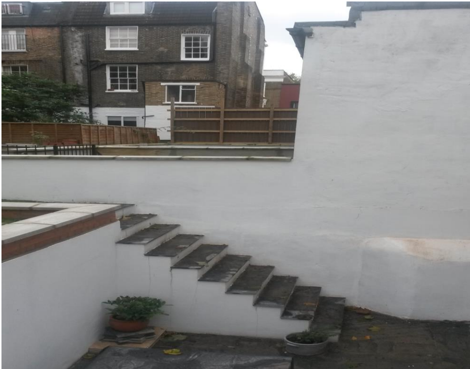
Photo 6: View of the existing basement lightwell to adjoining neighbour No.354 Caledonian Road and the extent of the two storey full width rear extension at No.352.
