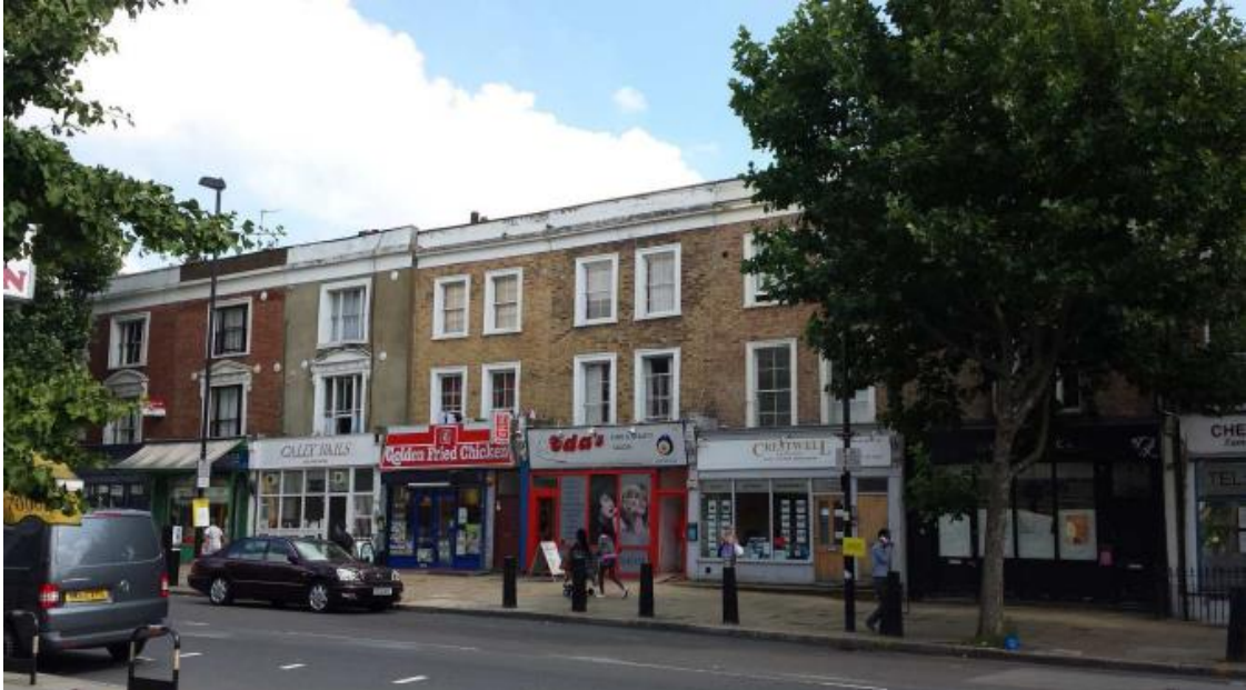
Image 2: Front Elevation of the application site and terrace at Caledonian Road
