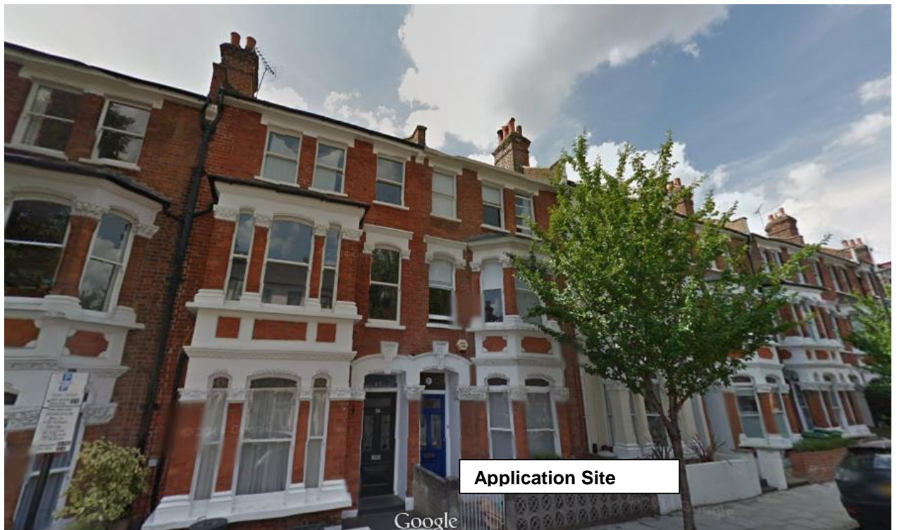
Photo 3: Existing front elevations along Calabria Road
