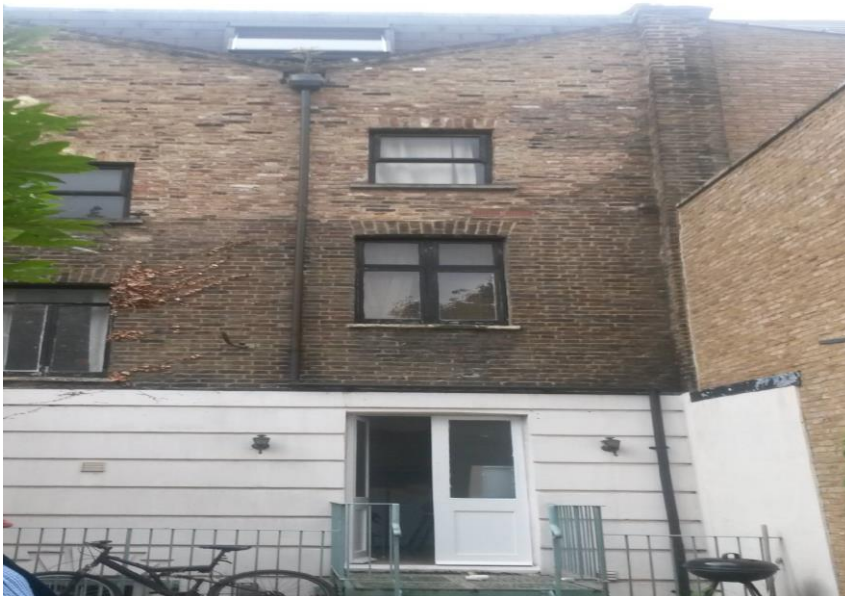
Photo 2: Rear elevation of the application property at garden level.
