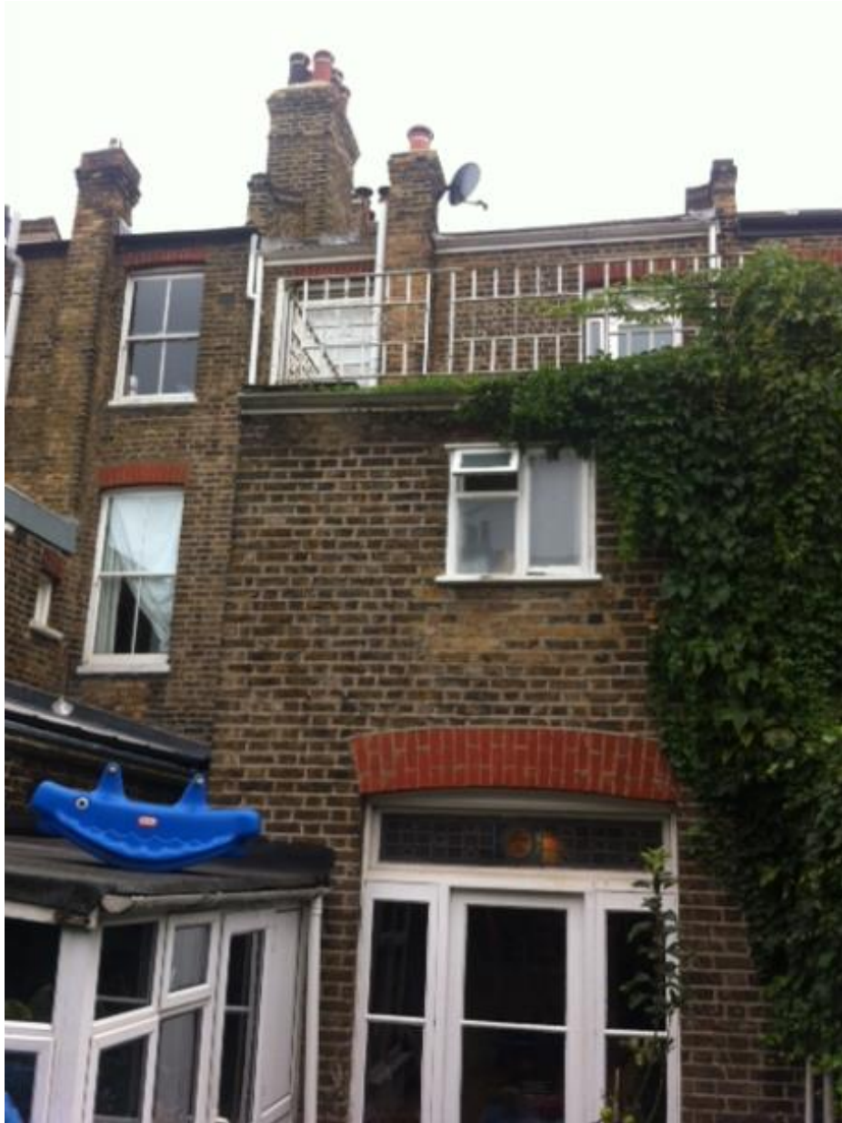
Photo 4: Rear elevation of application site (including existing roof terrace)
